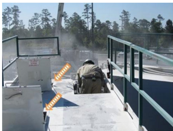
Figure 2. Sand mover operator at his work station on top of the sand mover, arrows point to the open thief hatches. Photo courtesy of Eric Esswein, NIOSH.
