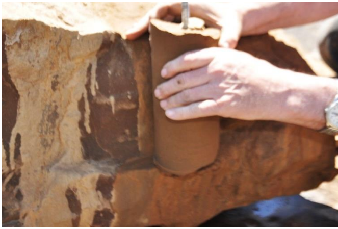
Fig. 26. Failure surface of core appears to match a cold joint.
