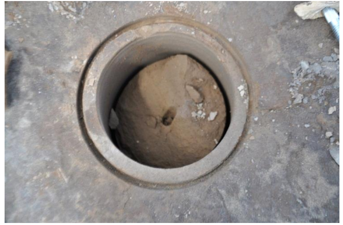
Fig. 23. Shear stress failure shown on the portion of test core remaining in the drill hole.
