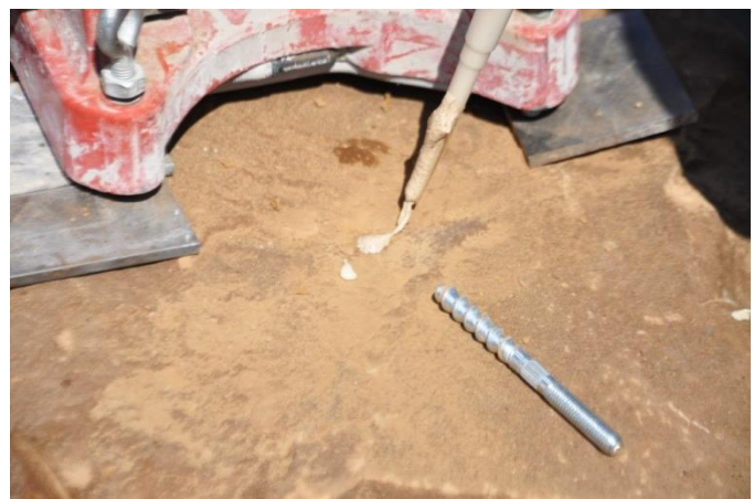
Fig. 12. Pilot hole filled with epoxy prior to insertion of pulling bolt.
