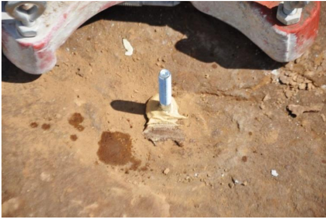
Fig. 13. Pulling bolt placed in the epoxy and cured overnight.
