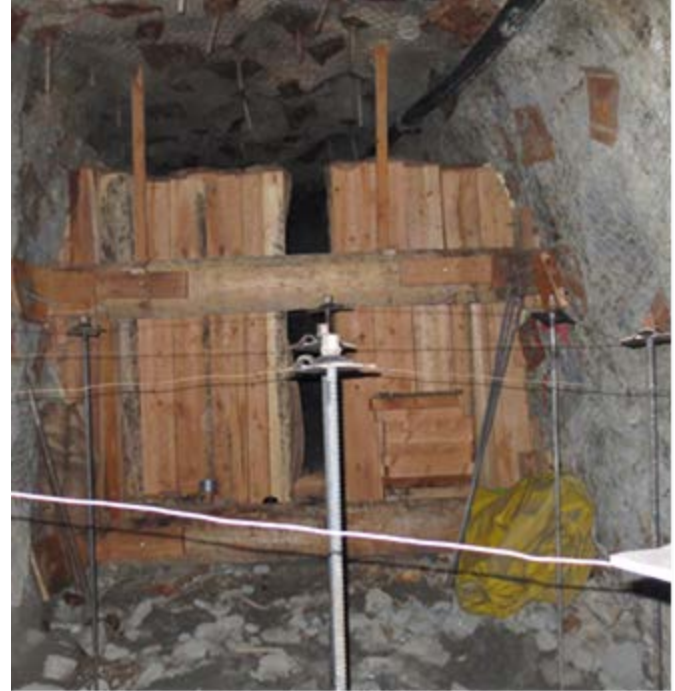
Fig. 2. Preparing a stope for backfill.
