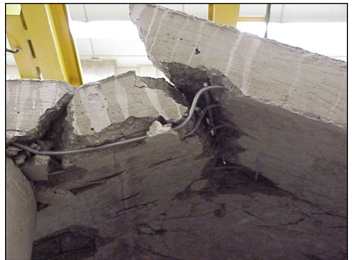
Figure 14. HEHD panel test sample with exposed wire mesh.
