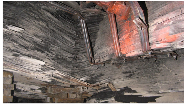
Fig. 5 Cutter roof failure of a weak shale rock at the roof-rib intersection
