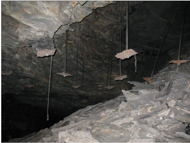
Fig. 11 Photograph showing how moisture-sensitive rock unraveled between bolts and fell to the ground
