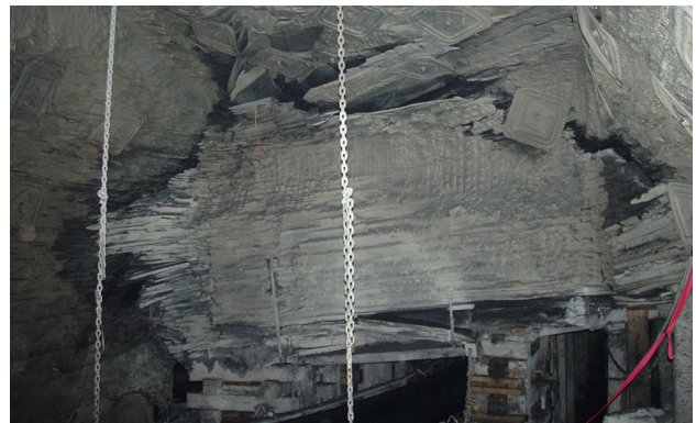
Fig. 6 Cutter failure that caused detached block, leading to a dead load of rock resting on support
