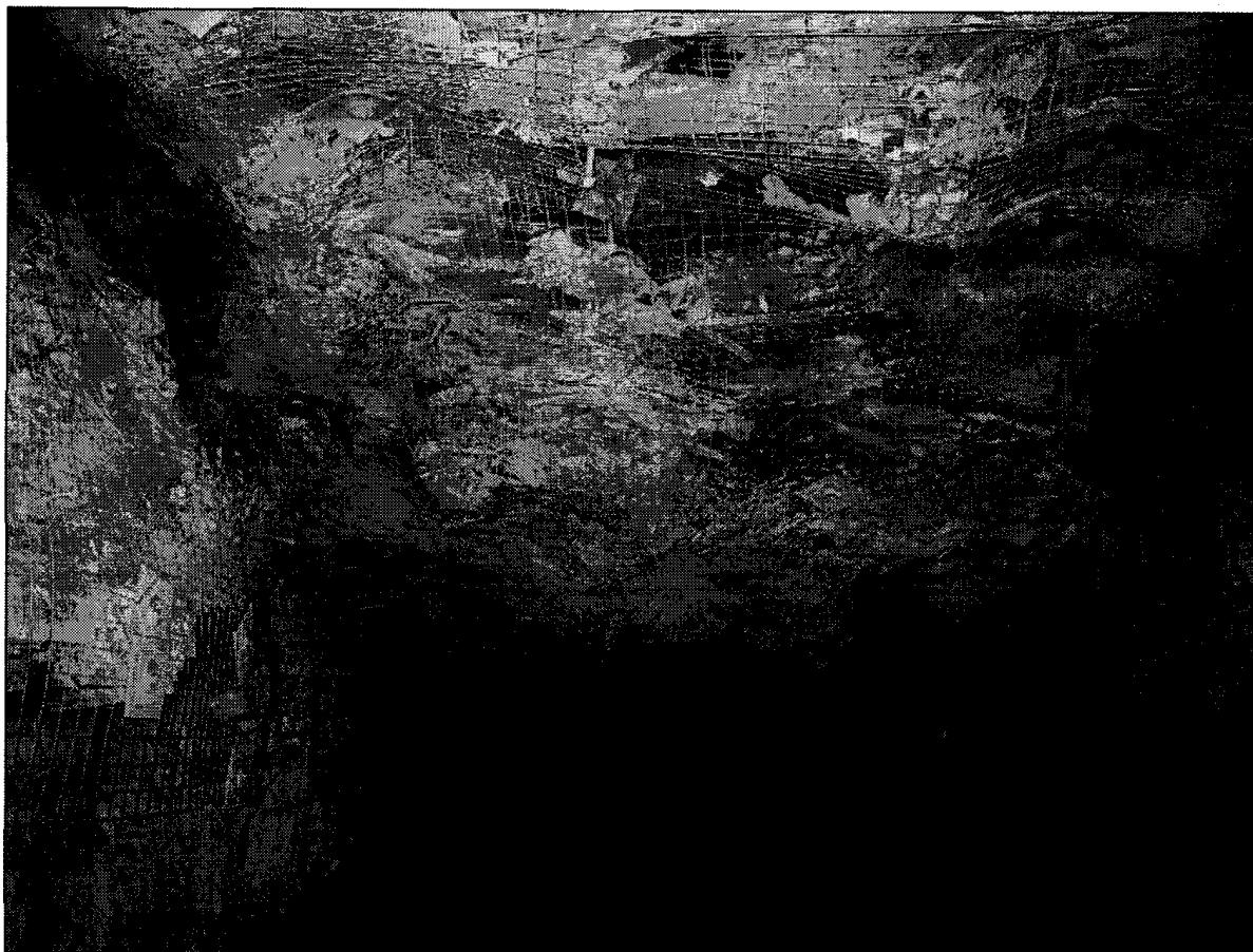
Figure 12 – Example of roof screen used to control deteriorated roof.
