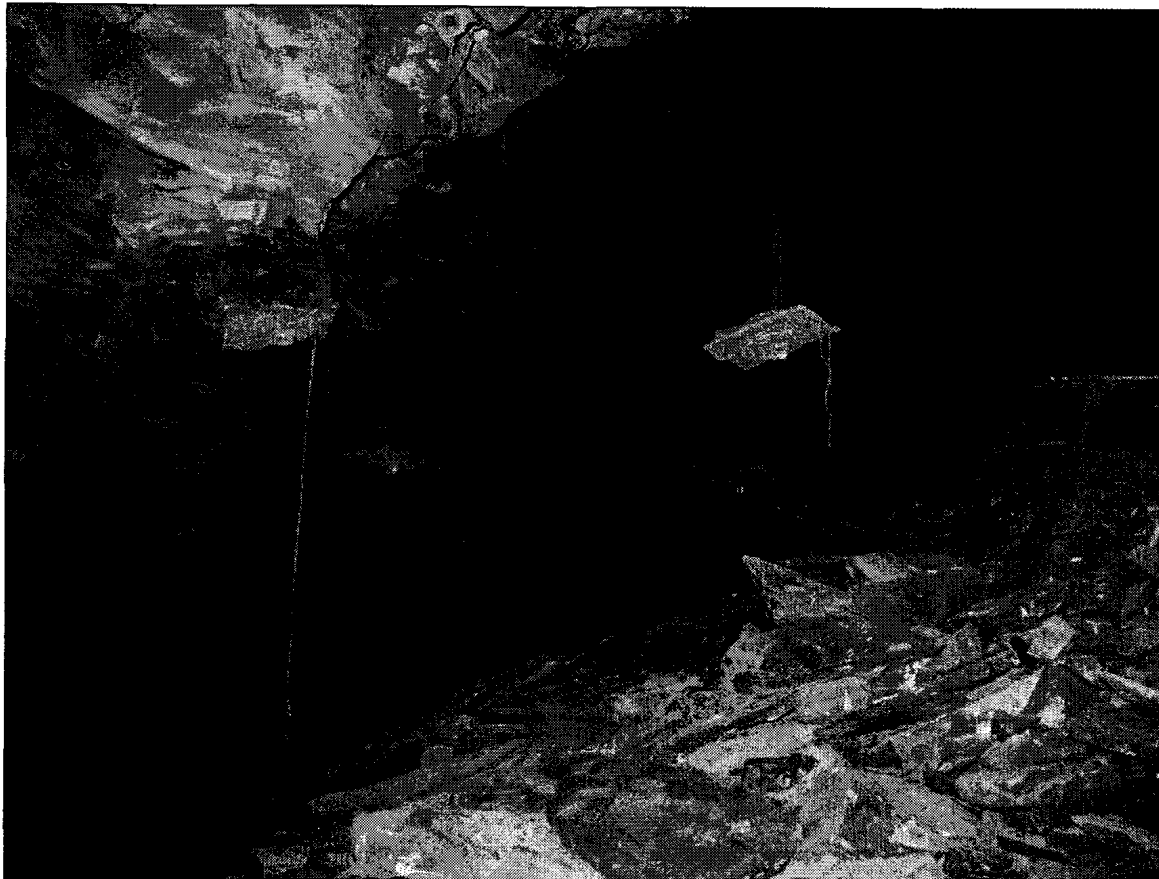
Figure 10 – Photograph showing how moisture-sensitive rock unraveled between bolts and fell to the ground.
