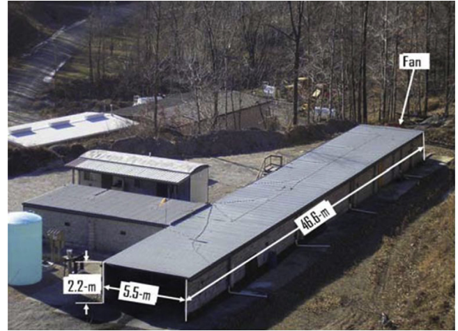
Fig. 1 – NIOSH Fire suppression facility.
