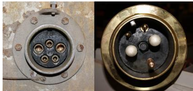
Fig. 7. Five-pole battery cable connectors.
