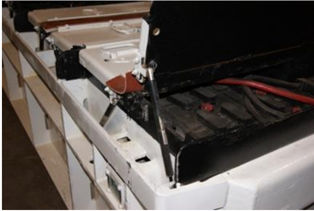
Fig. 5. Battery assembly with a pneumatic lift assist.
