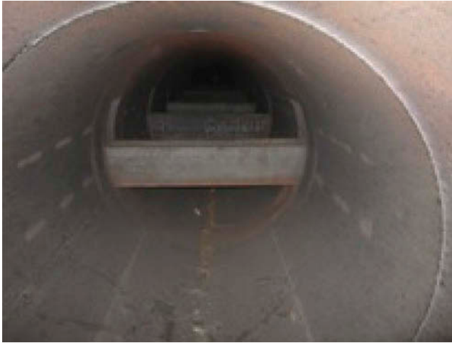
Figure 6 New baffle system using 200 W × 100 H sections.
