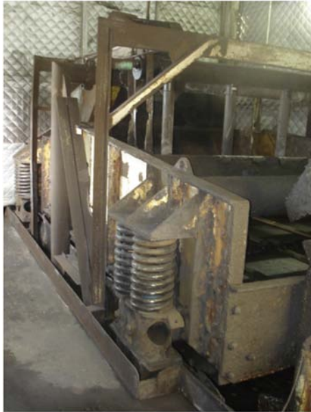
Fig. 19—Barrier wall surrounding the screen.
