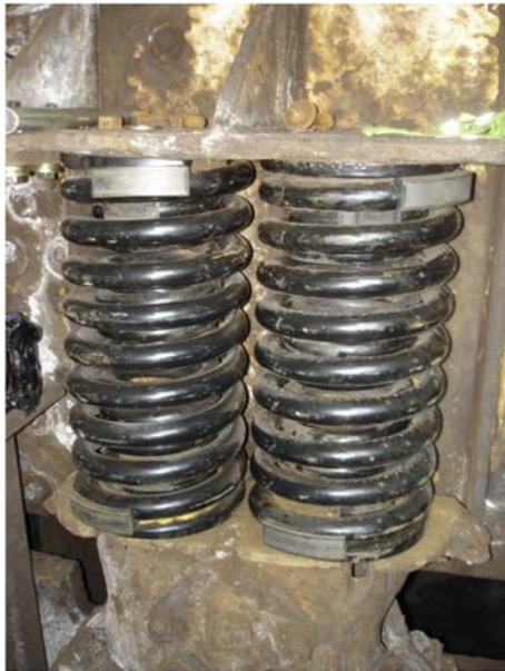
Fig. 21—Spring inserts in place and springs installed on the vibrating screen.
