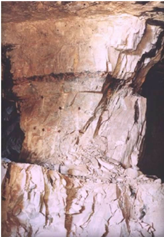
Fig. 6 Pillar impacted by large angular joints along the edge of bench mining showing sections of the pillar that fell away during bench mining (photo by A. T. Iannacchione)
