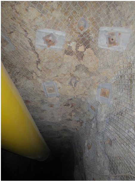
Fig. 10 Surface extensional fracturing due to horizontal closure in a back composed of CPB
