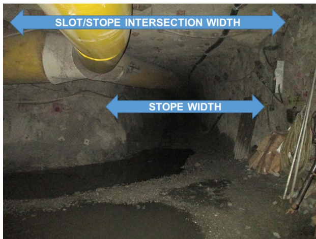
Fig. 8 Photograph in 6350 level (1935 m below shaft collar), 32-slot intersection looking toward 12-stope east and showing difference in span width for intersection and undercut stope
