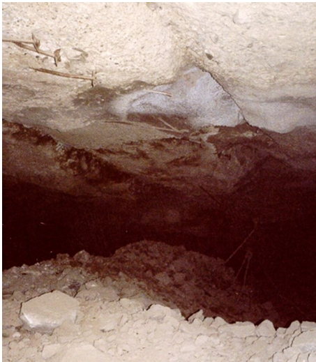
Fig. 21 View of final 13.7-m (45-ft) wide backfill span from the TR 4135 access (July 2001)
