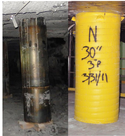
Fig. 5 Example of a can type support (left) and pumpable crib (right)
