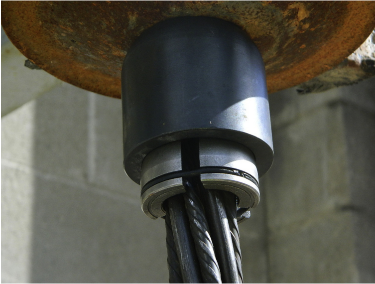
Figure 10.21 Hollow-cable bolt.
