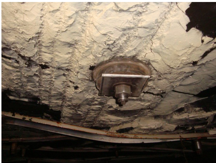
Figure 10.15 Tensionable cable bolt with nonrotation sleeve installed with a pressure pad to determine initial and subsequent loads.
