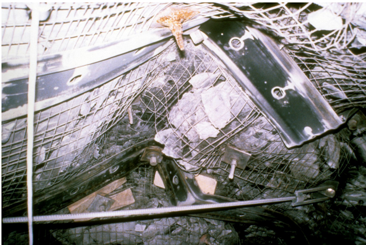
Figure 10.13 The roof is “folded” as illustrated in the bent heavy roof mats from the lateral movements and shear loading. The cable bolts installed in the mats are intact and continue to support the failed material.
