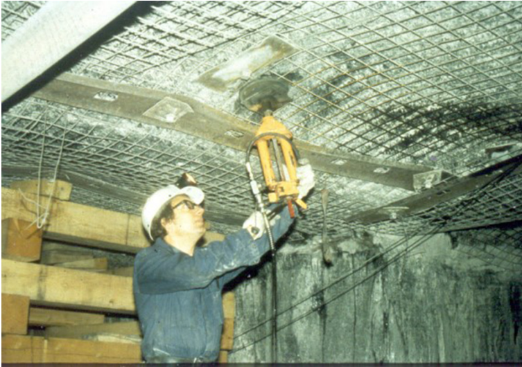
Figure 10.6 Post tensioning a cable after installation.
