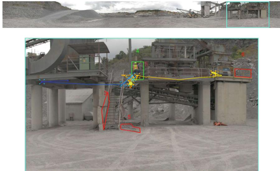
Fig. 2. Close-up view of a panoramic image from the mine plant showing an area with clustered hazards where only the highest-rated hazard was identified. Green ROIs indicate a hit; red ROIs indicate a miss. Each ROI is also identified with a unique ID number. The scan path line is color-coded from cool to warm colors before and after the button press. The click icons indicate fixations and the yellow dot represents the fixation location associated with the button press.
