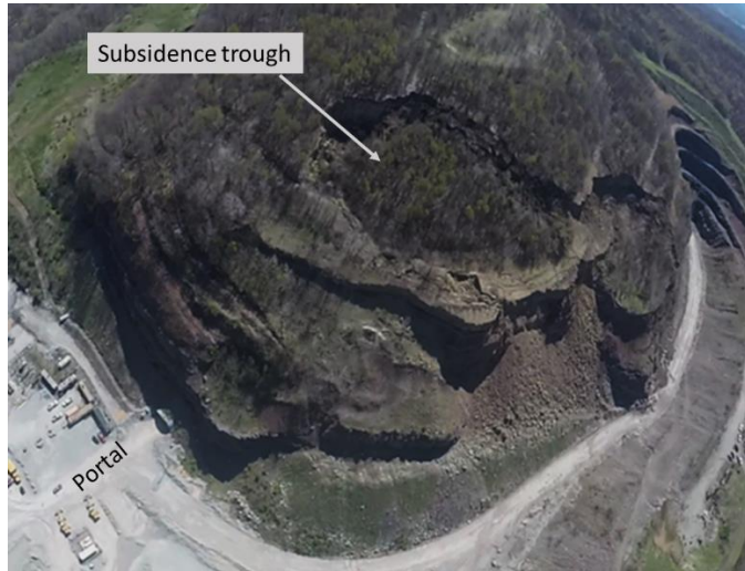
Figure 1. Aerial view of the mine showing extent of surface subsidence associated with the collapse of the pillars.
