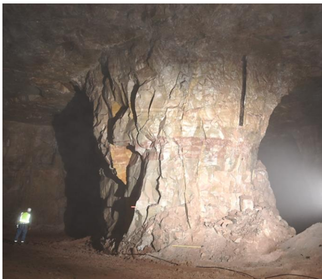
Figure 6. Pillar adjacent to collapsed area affected by angular jointing.
