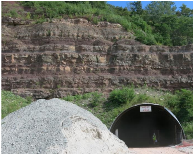
Figure 2. Main portal entering the mine with Mauch Chunk beds exposed in the highwall.
