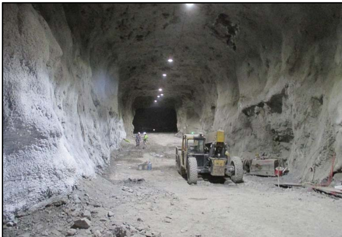
Figure 2. Competent ground away from ore bodies can allow for very large excavations for permanent infrastructure.
