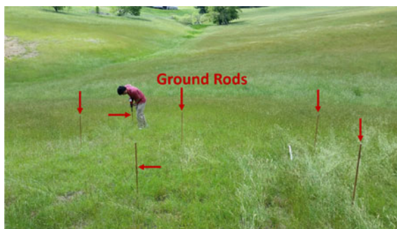
Fig. 7. Installing rods in a single earth electrode location.
