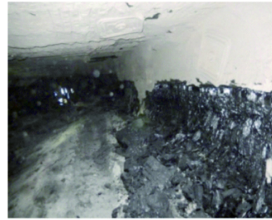
Fig. 20. Rib sloughage at the barrier side in the bleeder entry of Panel II in the lower seam.
