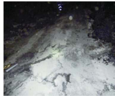
Fig. 21. Floor heave in the bleeder entry of Panel II in the lower seam.
