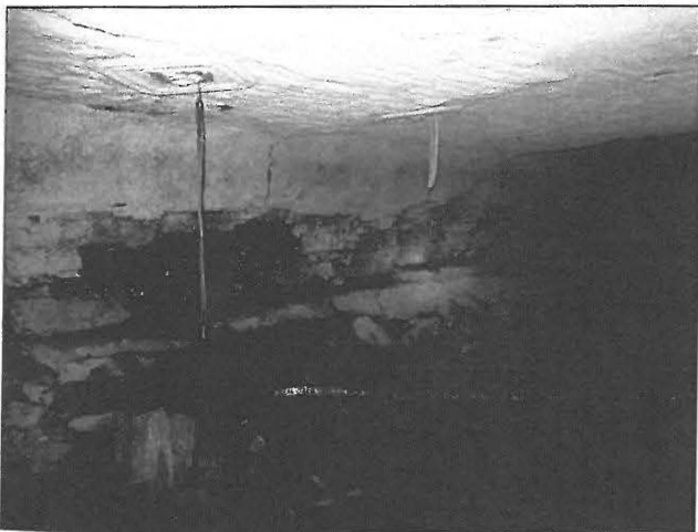
Figure 15. Rib sloughage outby the pillaring line during retreating in the upper seam.
