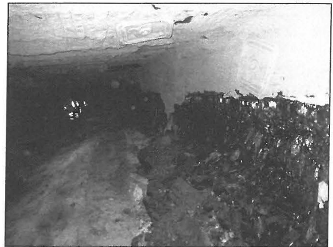
Figure 20. Rib sloughage at the barrier side in the bleeder entry of panel II in the lower seam.
