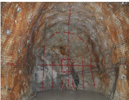
Figure 13. The buffer row design painted on the face.
