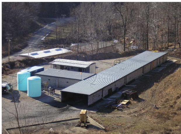
Figure 1 — Fire suppression facility.
