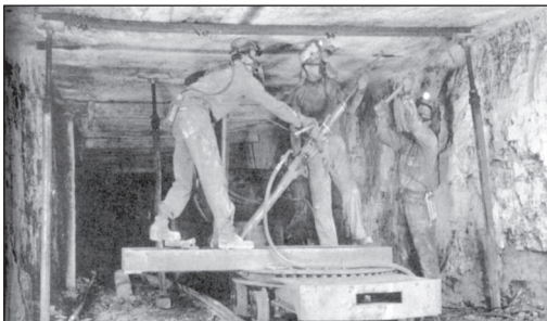
Figure 8. Dry drilling using respirators for dust protection
