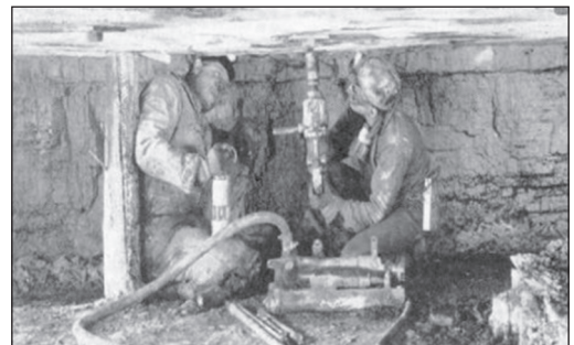
Figure 6. Installing roof bolts with a hand-held stopper drill
