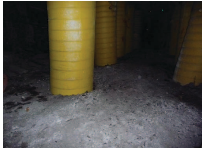
Figure 12. Floor heave developed during first panel mining from the side abutment at Mine B.
