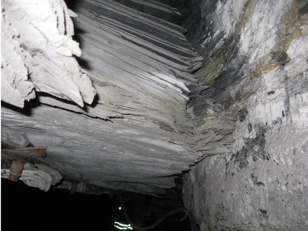
Figure 15: Cutter roof in thick shale roof sequence.
