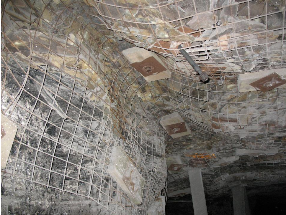
Figure 32: Rib and corner screening controls rib line guttering.
