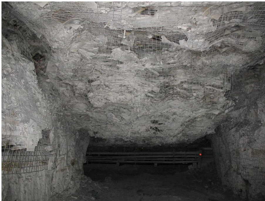
Figure 29: The rubbleized roof is effectively controlled by roof screen.
