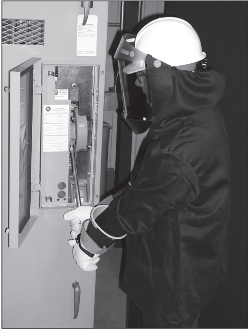
Figure 5. Appropriate arc flash personal protective equipment demonstrated by NIOSH researcher
