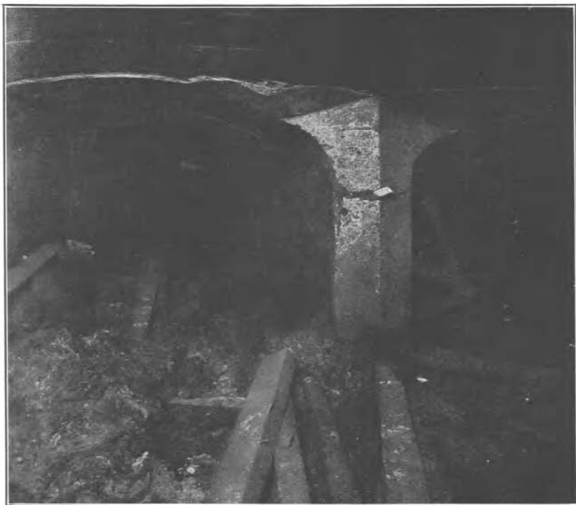
B. JUNCTURE OF GALLERY ENTRY AND AIR COURSE, SHOWING BROKEN REINFORCED CON- CRETE CORNER WITH CURTAIN AND WOOD IN THE CREVICES.
