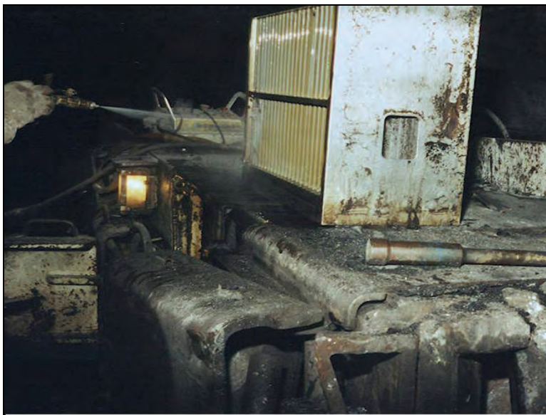
Figure 4-8.—Cleaning the demister with a water nozzle.
