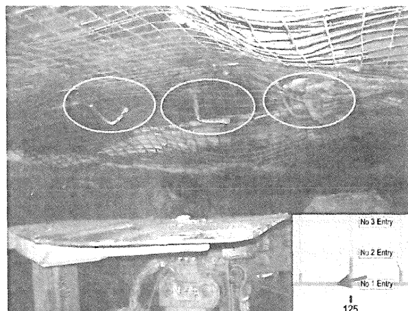
Figure 5. Damaged roof bolts in No. 1 entry after August 6 accident resulting from northern movement of southern barrier. Mesh shown was installed during rescue operations, over damaged original bolts. Camera view is indicated by arrow in index map insert (after Gates et al., 2008).
