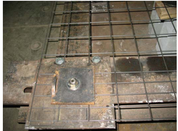
Figure 8. Wire configuration for 8-gauge screen with two additional reinforcing wires at each end of the screen. There are three transverse wires under the bearing plate.
