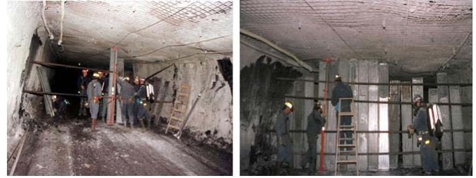
Figure 4. Construction of a Kennedy steel panel stopping in No. 2 entry.
