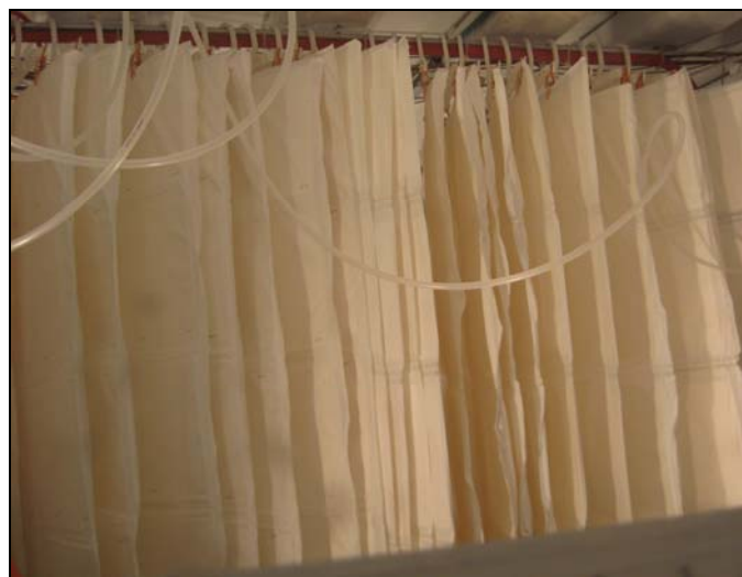
Figure 4. Passive lithium curtains for scrubbing carbon dioxide.
