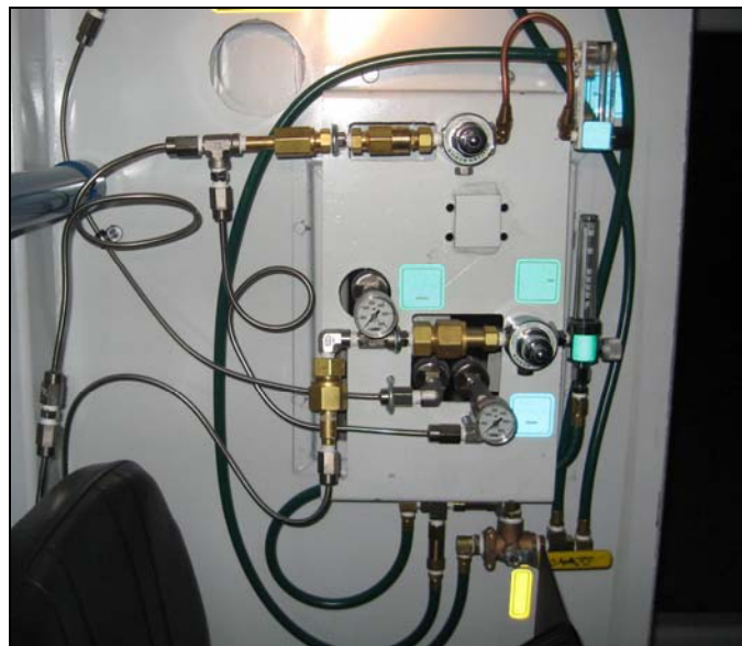
Figure 3. Example of oxygen supply system in a refuge chamber.
