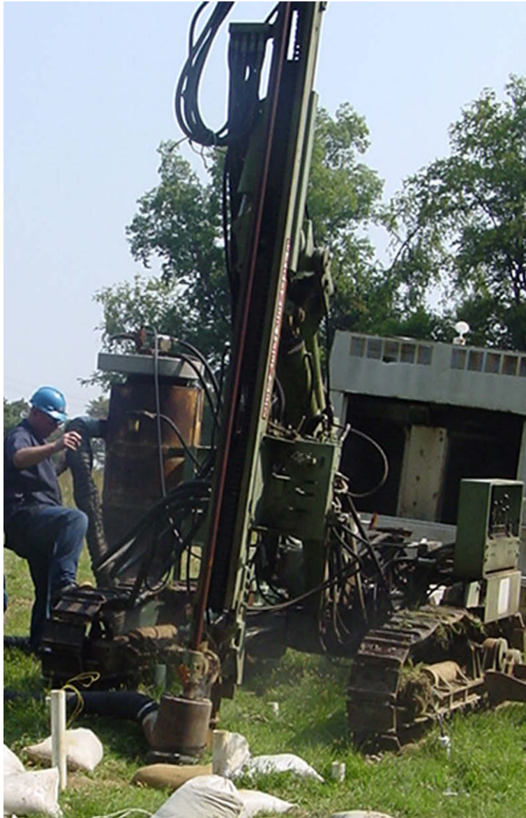
Fig. 5. Negative pressure application using the drill rig dust collection system.
