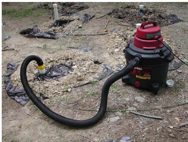
Fig. 3. Negative pressure application using a Shop-Vac.
