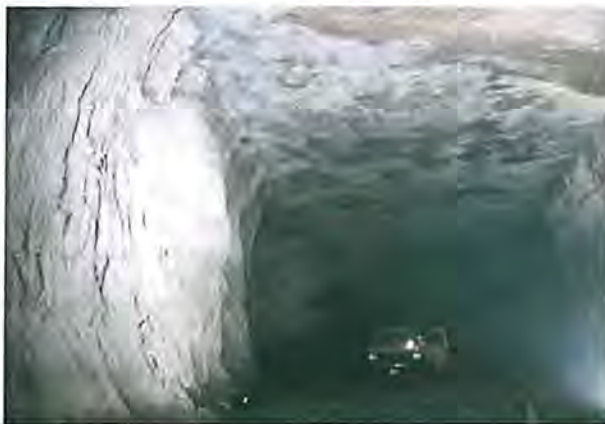
Figure 5. Example of rib slabbing and resulting concave pillar ribs that can initiate when average pillar stress exceeds about 11% of the UCS.
