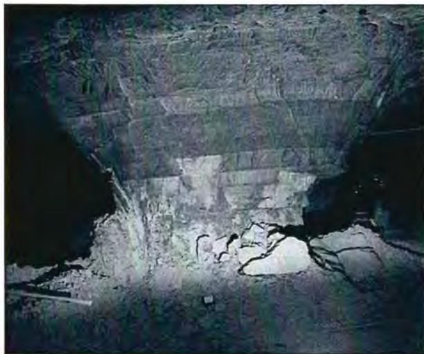
Figure 2. Pillar that has an original width-to-height ratio of 1.7 failed by progressive spalling. Thin weak beds are thought to have contributed to the failure. The average pillar stress was about 11% of the UCS prior to failure.
