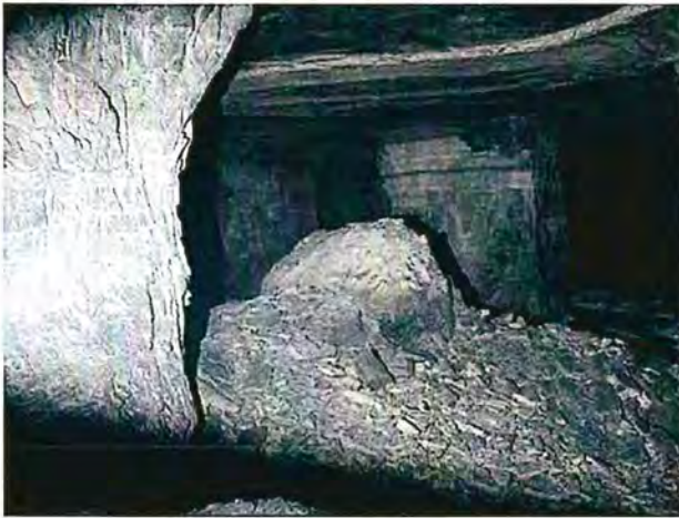
Figure 1. Remaining stump of a collapsed pillar in an abandoned area. Thin weak beds in the pillar and moist conditions are thought to have contributed to the failure. The width-to-height ratio was 0.82 and average pillar stress about 11% of the UCS.
