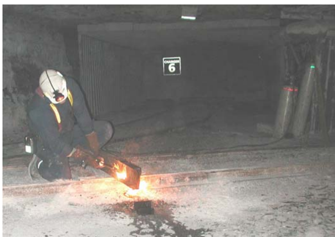
Figure 10. Flame cutting of a piece of rail.
