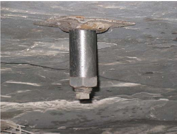
Figure 8. A "Ker-Thob" is used to re-establish plate contact with the roof and maintain roof bolt integrity.
