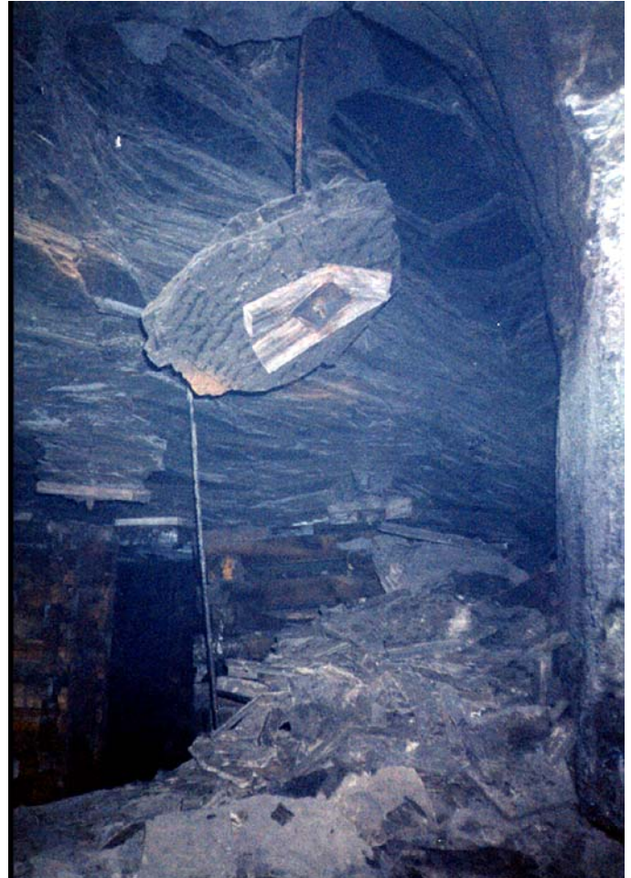
Figure 9. Severe guttering due to horizontal stress.
