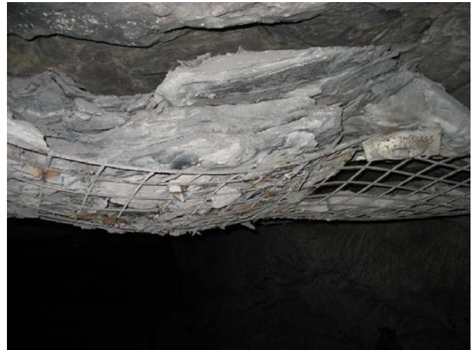
Figure 12. Roof screen loaded with rock.
