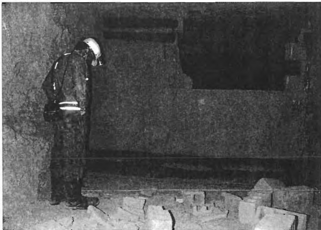
Figure 2. Ventilation stopping partially destroyed by explosion pressure.
