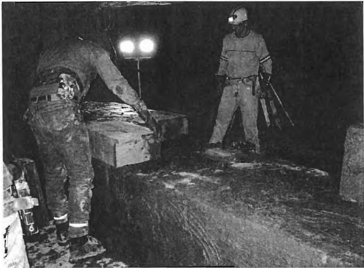
Figure 5. Construction of a mine seal.
