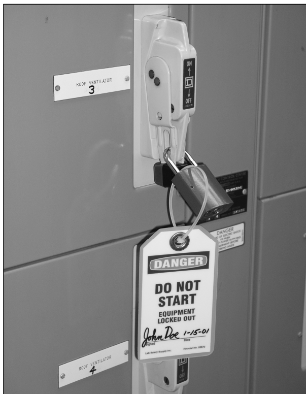
Figure 2. A properly applied lock and tag. Note that the tag cannot be easily removed, contains the name of the person who applied it, and the date of the work.
