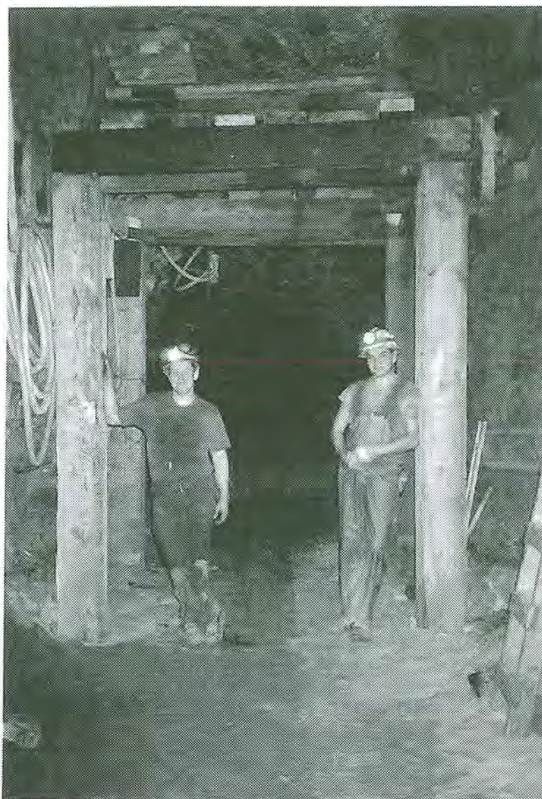
Figure 2: Traditional timber sets for hardrock applications.
