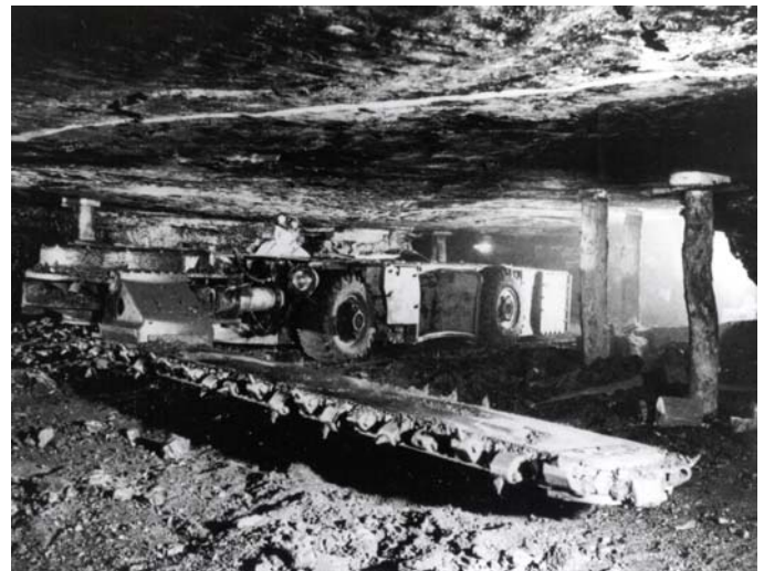
Figure 4. Jay boom cutter used in conventional mining.
