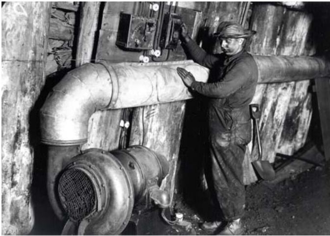
Figure 5. Auxiliary fan used to provide fresh air to the face.
