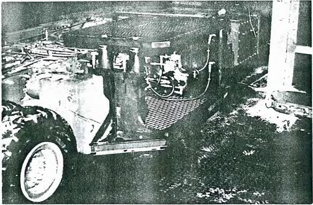
Figure 7. Canopy Trial Installation on Joy 16RB Cutter
