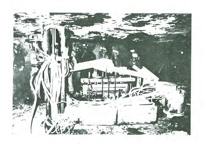
FIGURE 16. Automated roof bolting machine (Bureau of Mines, U. S. Department of the Interior).
