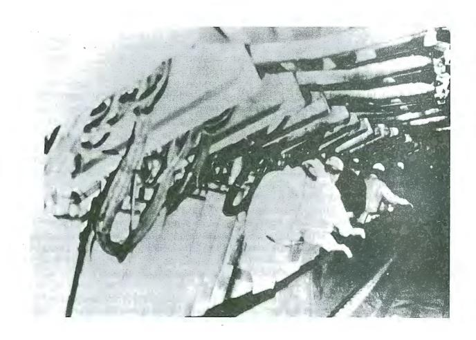
FIGURE 17. Shield-type supports being tested by the Bureau in Kaiser Steel Corporation's York Canyon Mine, in Raton, New Mexico (Bureau of Mines, U. S. Department of the Interior).
