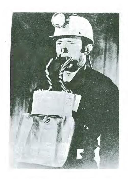
FIGURE 6. One-hour self-rescuer developed under a Bureau research contract by the Lockheed Missile and Space Company (Bureau of Mines, U. S. Department of the Interior).
