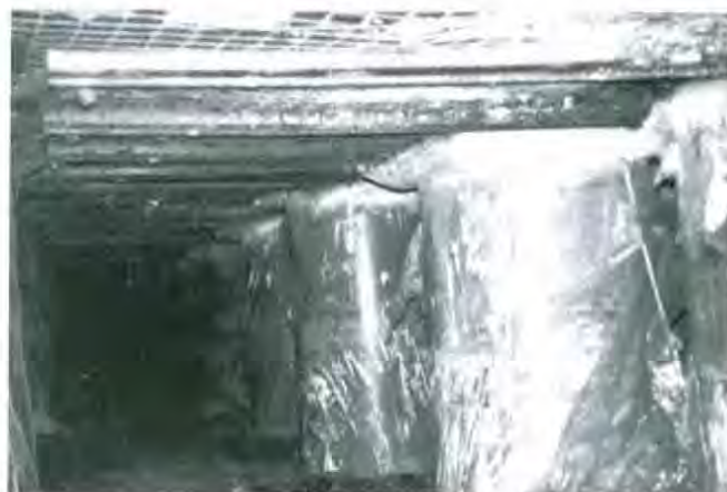
Figure 6 — Completed cribs, roof supports and instrumentation.
