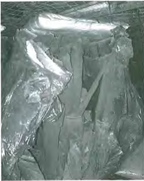
Figure 7 — Brittle crib failure prior to the longwall entering the recovery room.
