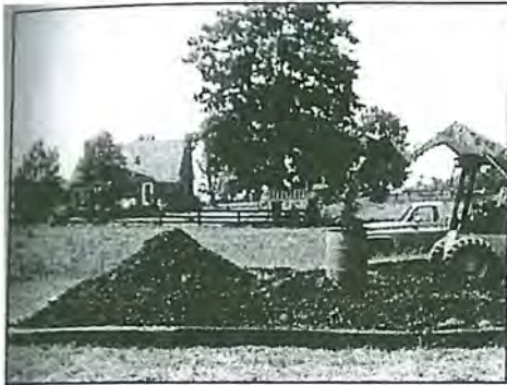
Figure 7.—Second perforated plastic barrel being covered with coal.
