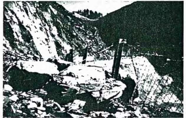
Figure 16. Catch fence installed to prevent loose rocks from traveling to the pit floor.
