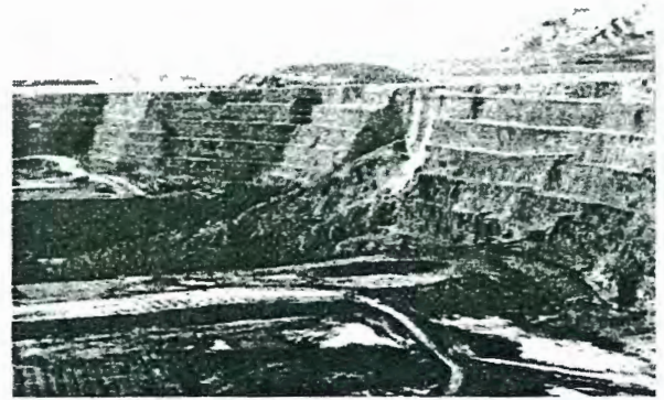
Figure 4. Massive slope failure at an open pit gold mine did not cause any injuries or accidents, but did cause significant production problems and high costs.
