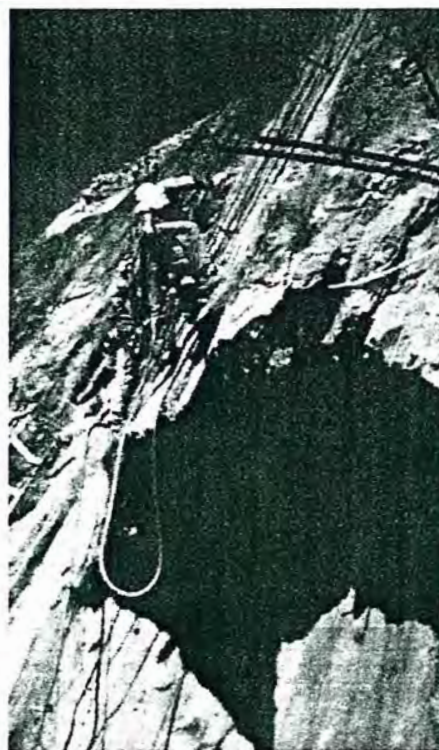
Figure 11. A worker suspended by mountain climbing gear is supporting a potentially unstable overhang with cable bolts.
