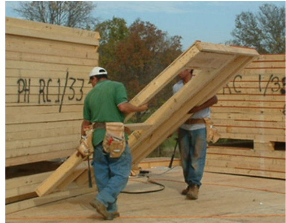
Fig. 1. Example of panelized residential construction.
