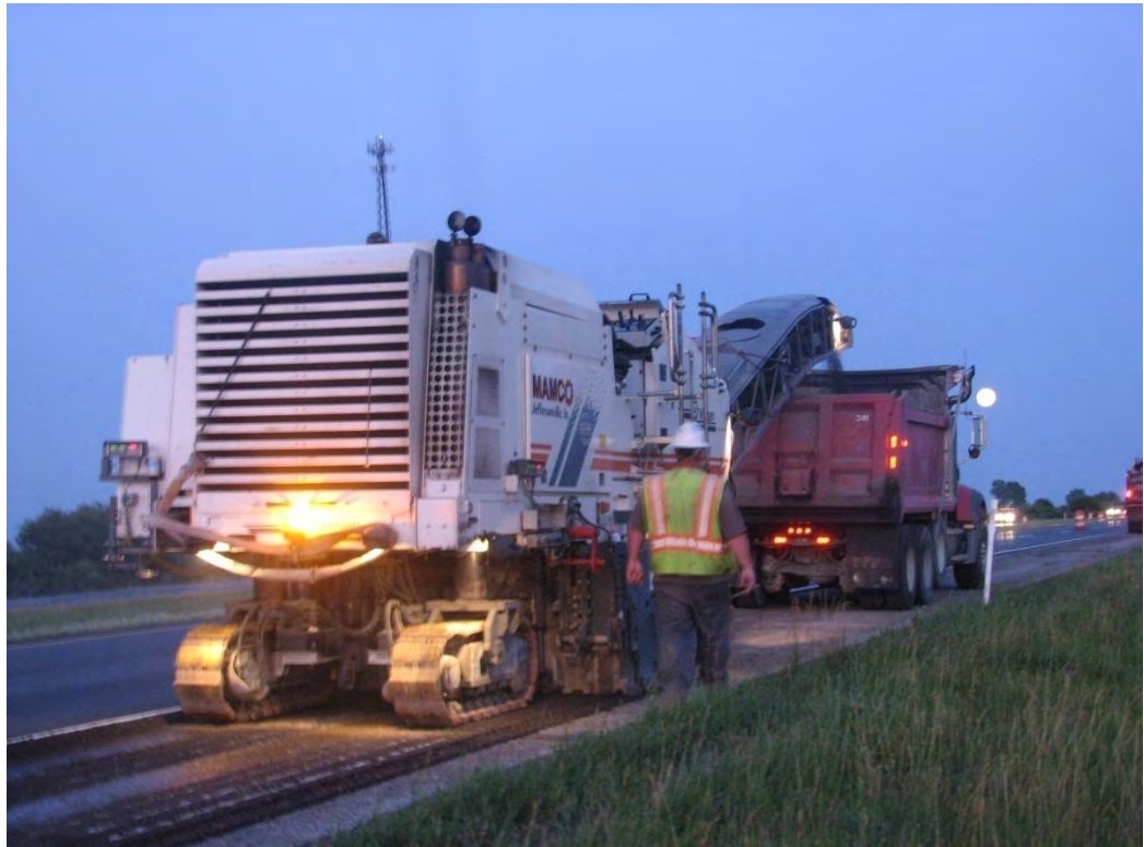
Figure 3.3: Milling of the asphalt pavement (photo taken during Site Visit # 3, I-65 S Mile Marker 150 on July 9, 2009)
