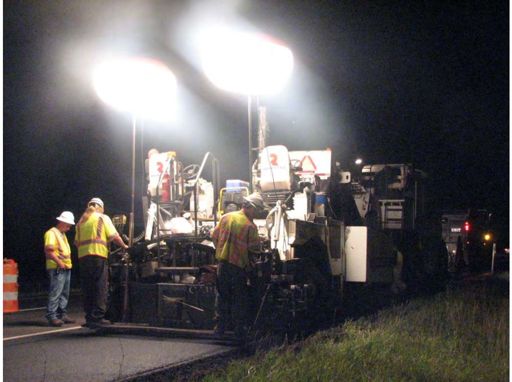
Figure 3.5: Laying the HMA coat on the pavement (photo taken during Site Visit # 3, I-65 S Mile Marker 150 on July 9, 2009)
