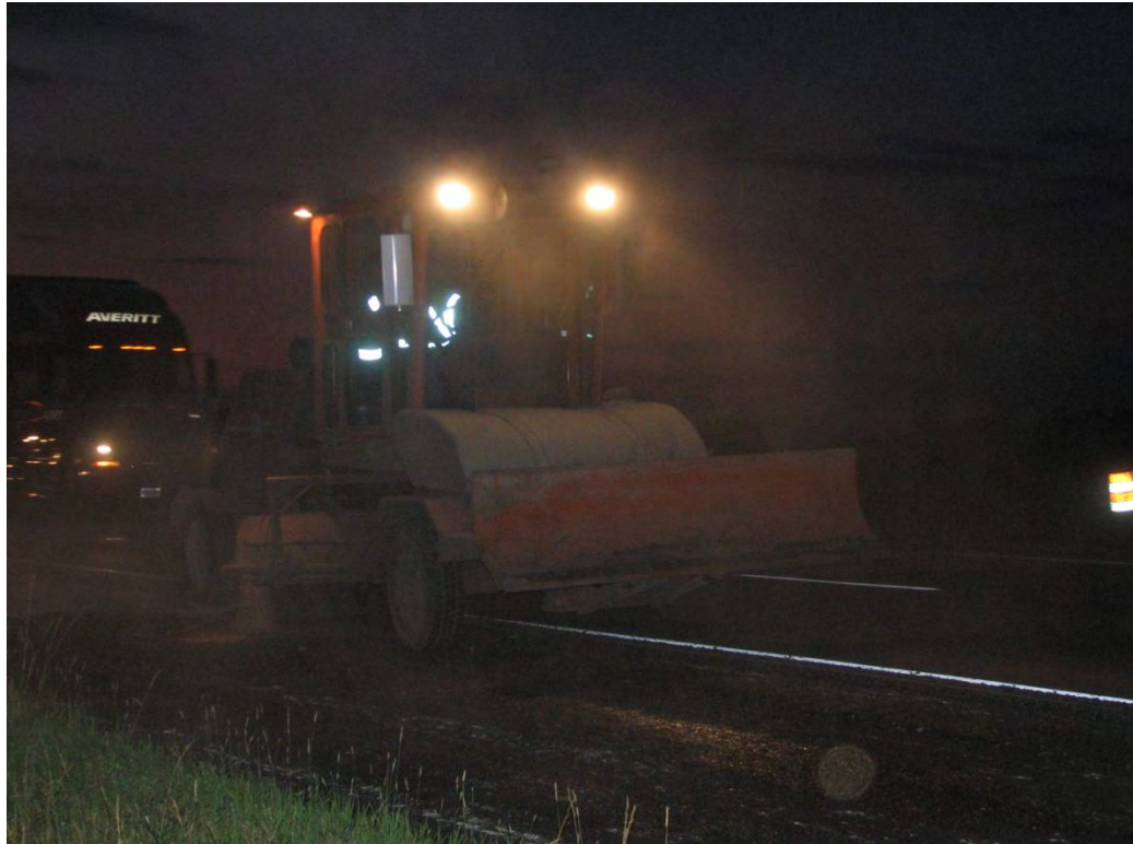
Figure 3.4: Sweeping the debris after milling is complete (photo taken during Site Visit # 3, I-65 S Mile Marker 150 on July 9, 2009)
