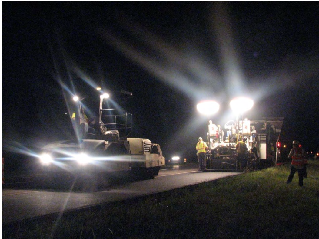
Figure 3.6: Compacting the HMA coat (photo taken during Site Visit # 3, I-65 S Mile Marker 150 on July 9, 2009)
