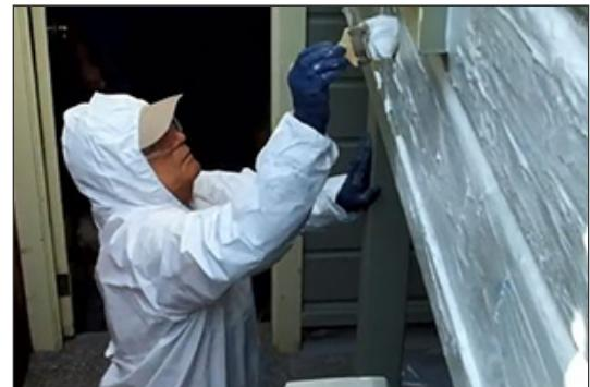
*Photo: A worker applies a safer paint removal product.*
