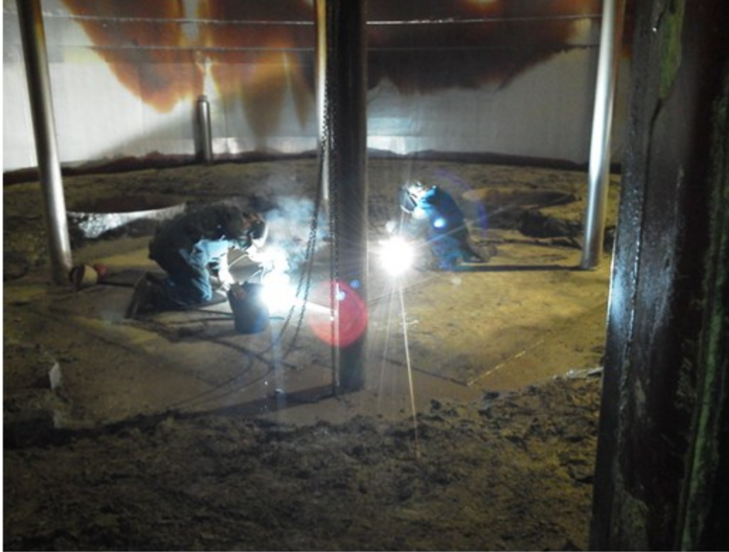
Figure 2: Individuals Performing SMAW in a Scrubber Vessel
