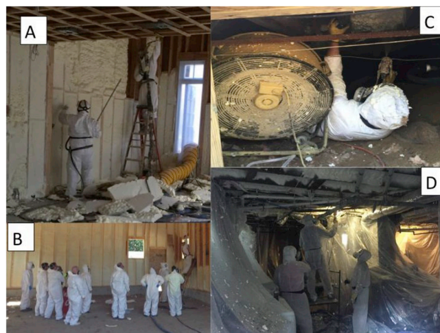
Fig. 1. Representative, illustrative pictures of insulation workers investigated in this study. A: SPF spraying (sprayer and helper) of a new construction home by a large contractor; B: Training on SPF application at a training center (new garage); C: Insulation of the 1st floor of an existing home by a small contractor; D: Insulation of the basement of an existing home by another small contractor.
